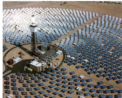
Solar Two, US Dept. Energy
