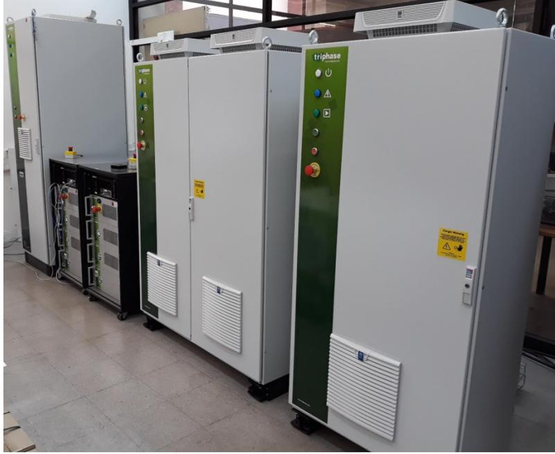
Figure 5.10: Experimental system based on five Triphase power converters, nominal powers 5-30kW (each one). They are configured to emulate the topology of Fig. 5.9.
